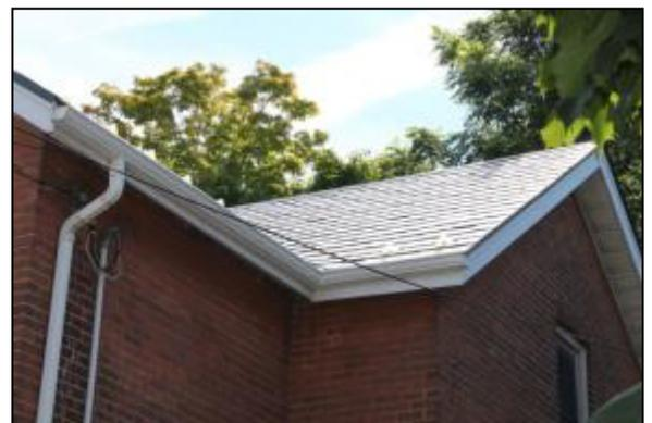
Composite roof materials may be an appropriate replacement material.
