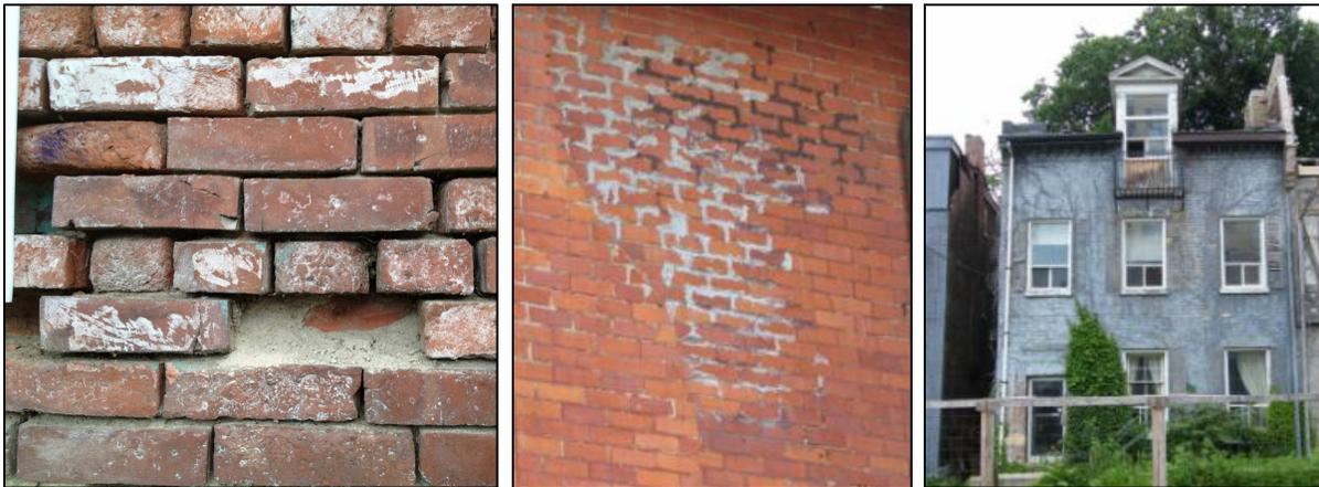
Masonry may need to be re-pointed over time to extend its lifespan and avoid damage. Care should be taken when re-pointing to match mortars and techniques (unlike the example in the centre). Painting of previously unpainted masonry surfaces is not permitted (as in the example on the right).
