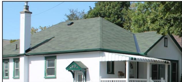
There are a variety of roof types within the District. Existing roof types shall be maintained. Many roofs have asphalt or metal shingles, which may be replaced in kind.
