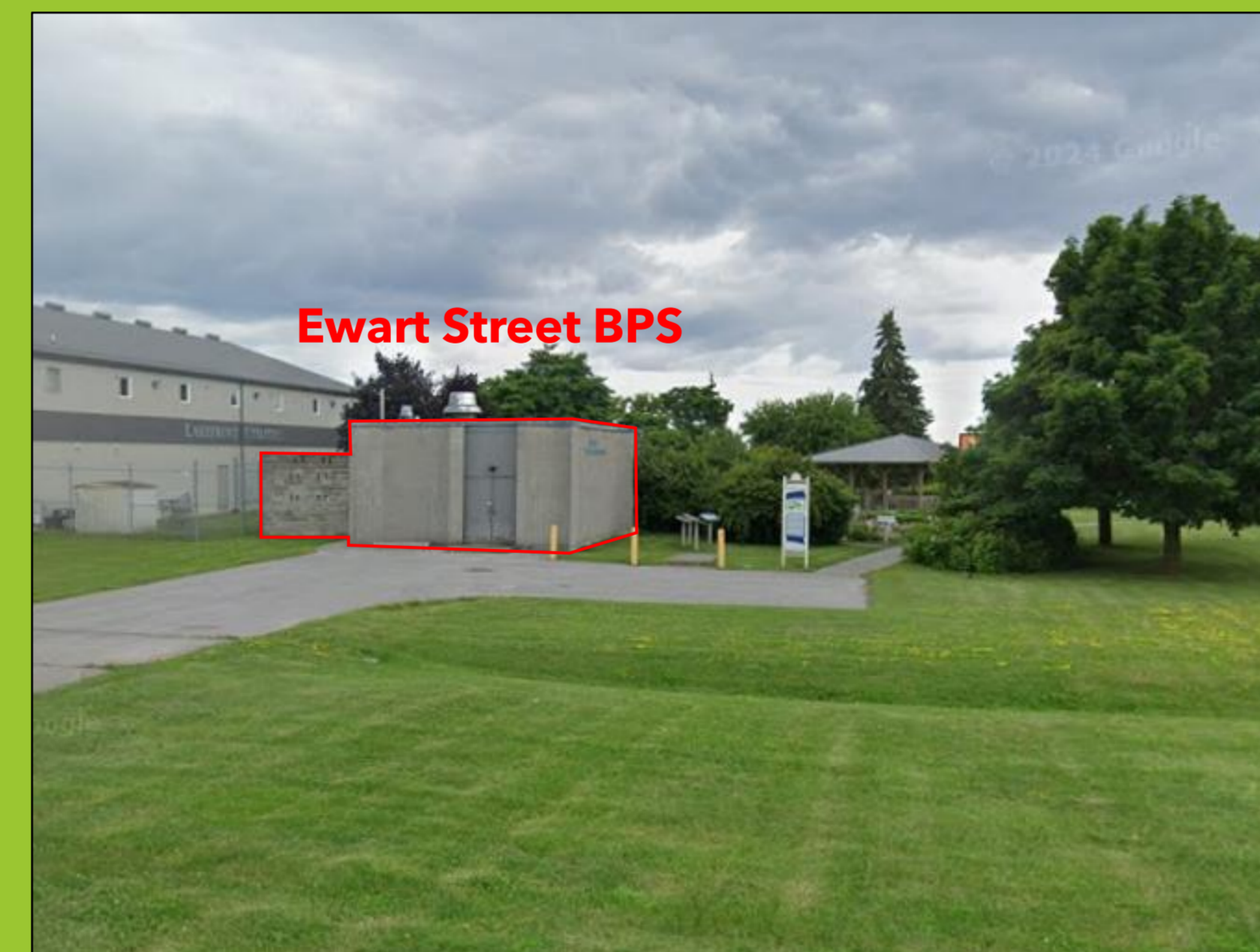
Existing BPS Facility at Ewart Street
