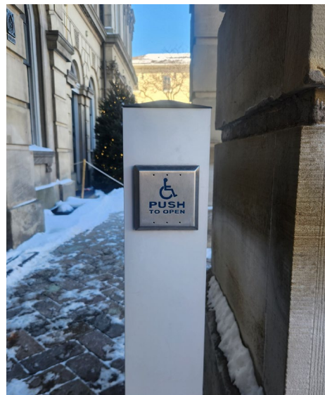
The new accessible door opener located outside the main doors at Victoria Hall.
