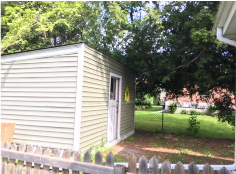
Photo 2: Looking North towards existing shed on the subject property, which will be removed to accommodate the proposed building addition within part of the footprint.
