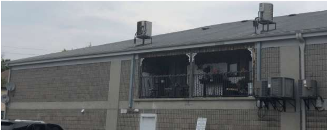
Figure 5: Existing condition of current asphalt roof looking north east.
