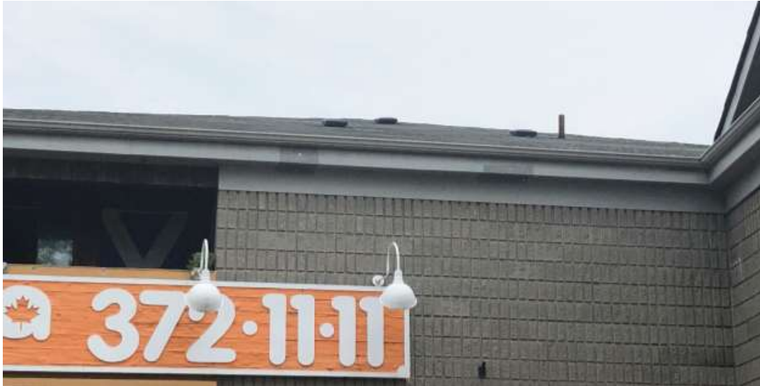
Figure 2: Existing Condition of current asphalt roof looking north
