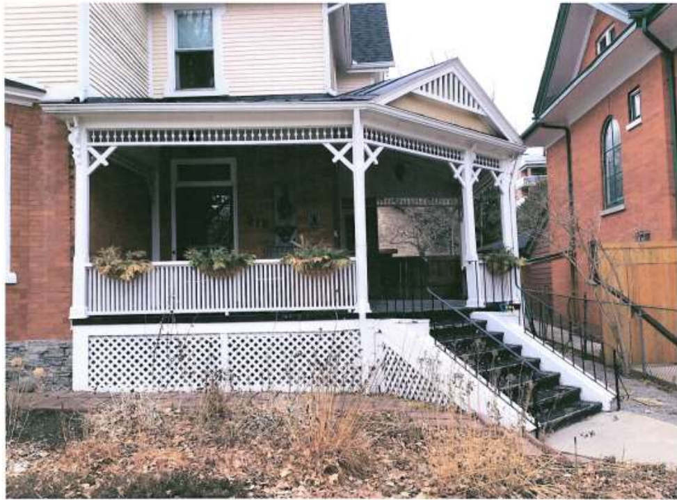
Figure 1: Existing porch at 216 Church St.
