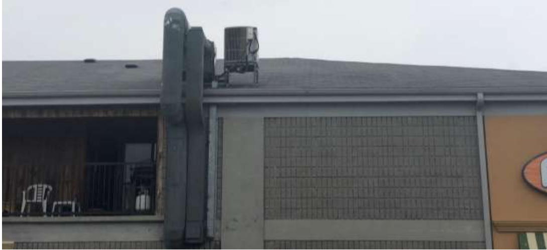
Figure 4: Existing condition of current asphalt looking east.
