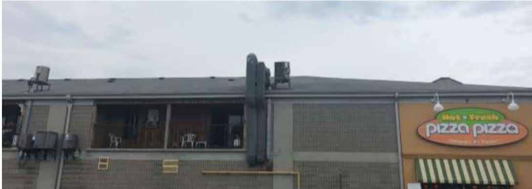
Figure 3: Existing condition of current asphalt roof looking east.
