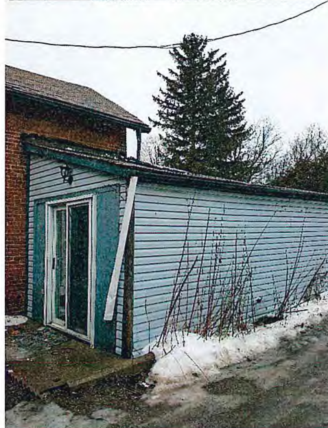
Above: Exterior of the modern addition/garage in a state of disrepair. Damaged eaves trough and roof. Removal of entire side addition.
