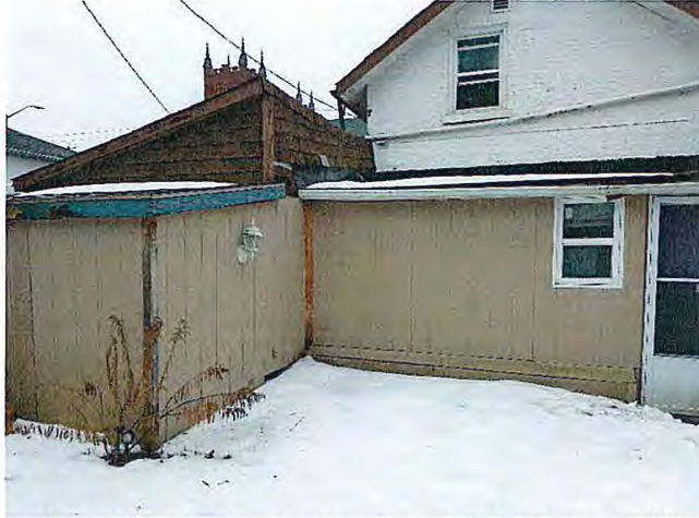
Above: Existing modern addition/garage structure. Removal of entire rear addition.
