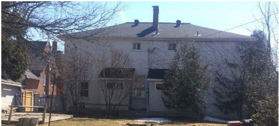
Figure 6: Rear additions to be demolished
