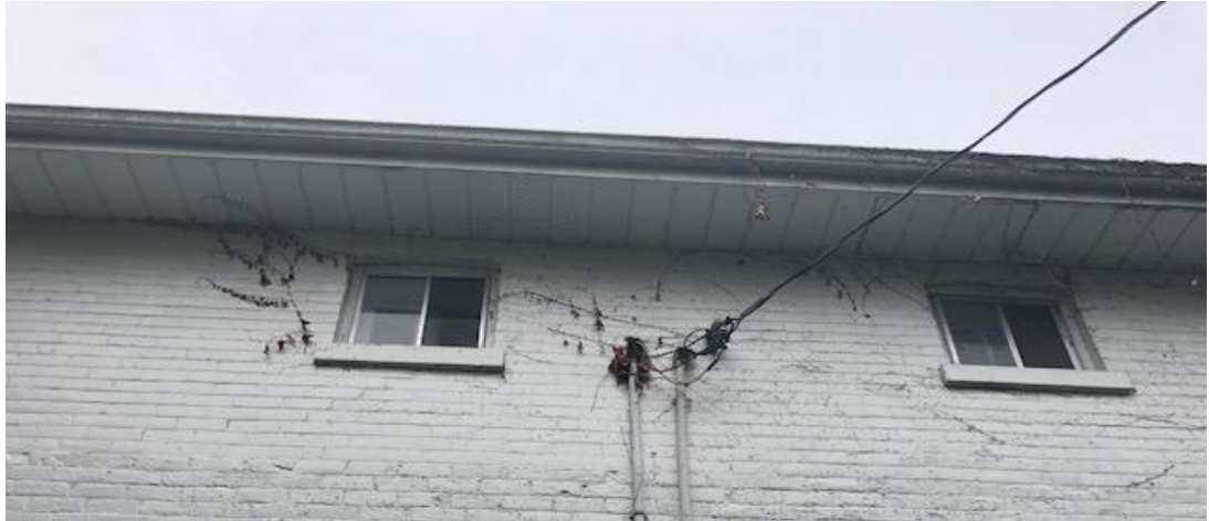
Figure 14: Exterior rear aluminum storms on upper floor bathrooms to be replaced on both 22 (on the left) & 24 (on the right) University Ave. W.
