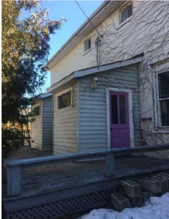
Figure 7: Rear additions to be demolished close up
