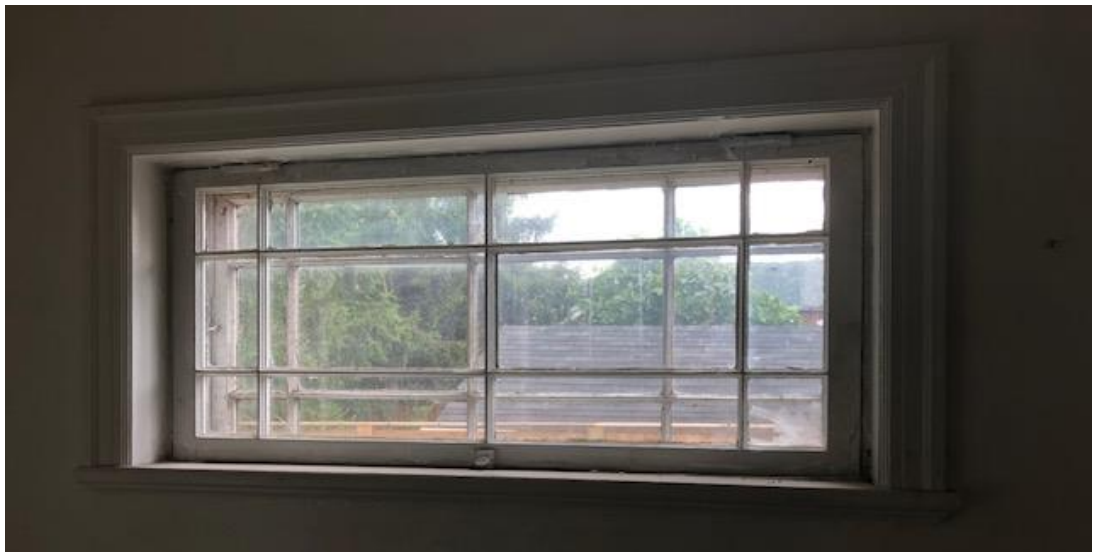
Figure 8: Current condition of the only surviving original window. Applicants will repair and maintain. (interior photograph). 22 University Ave. W
