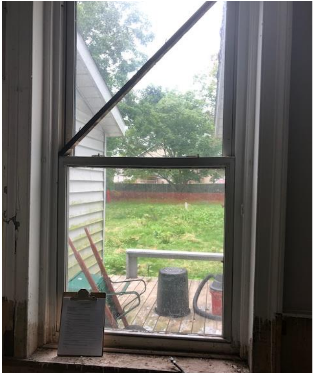
Figure 13: Rear west window of 22 University Ave. W to be replaced (42" x 81") vinyl for vinyl. Window is broken, will not stay open. Notice the sill, there was a countertop installed with no flashing.
