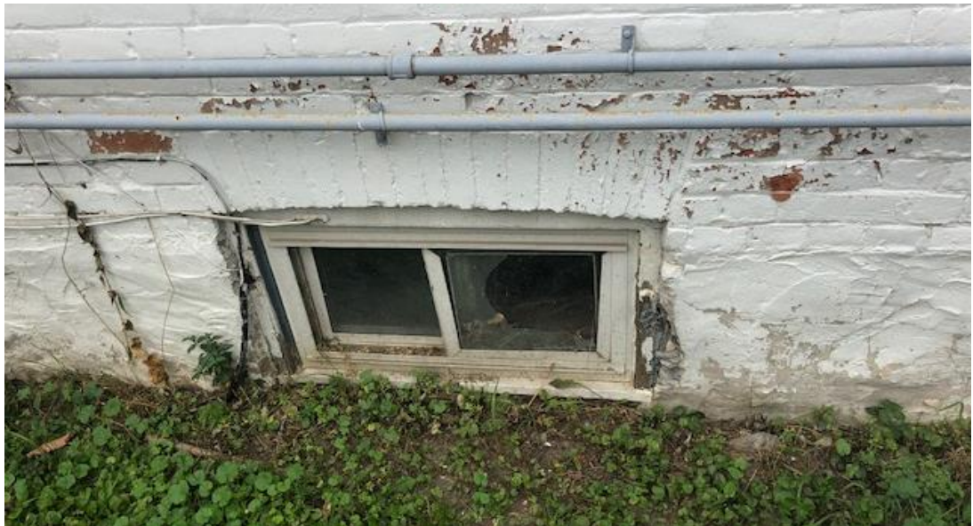
Figure 12: Basement window (exterior) to be replaced (49" x 22") vinyl for vinyl. Product information above.
