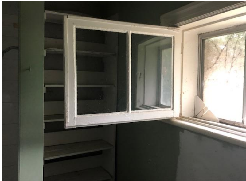
Figure 17: Interior original wood window at 24 University Ave. W, single opening. Notice the difference from above (fig. 14 &15). Aluminum storm to be replaced.
