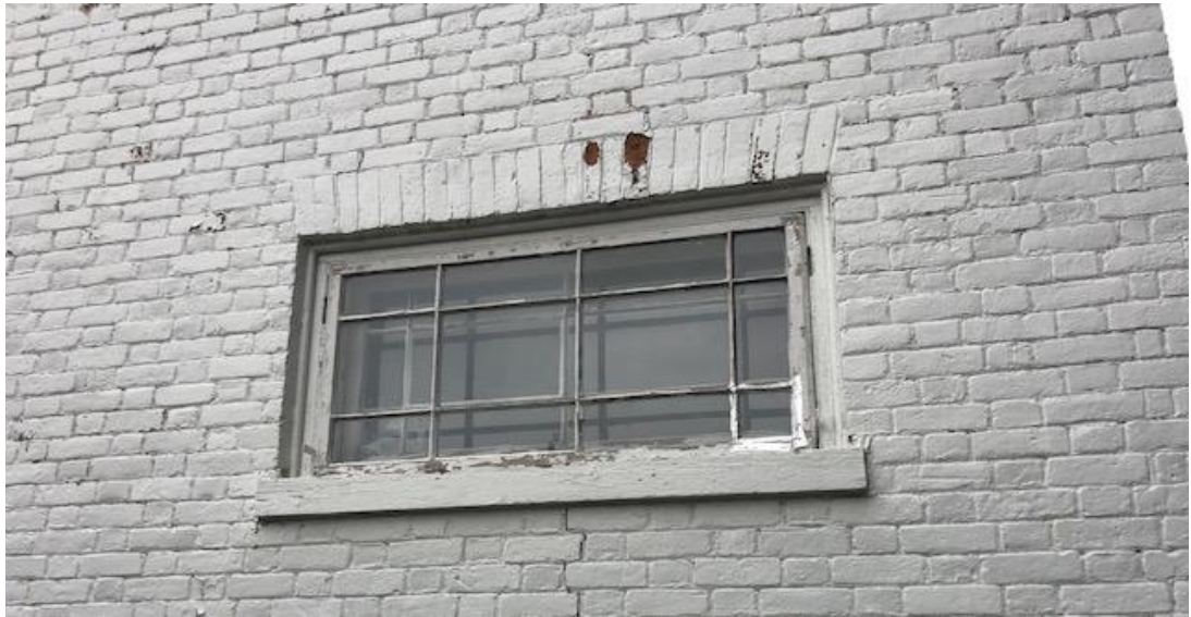
Figure 9: Exterior photograph of the only surviving original window. 22 University Ave. W.
