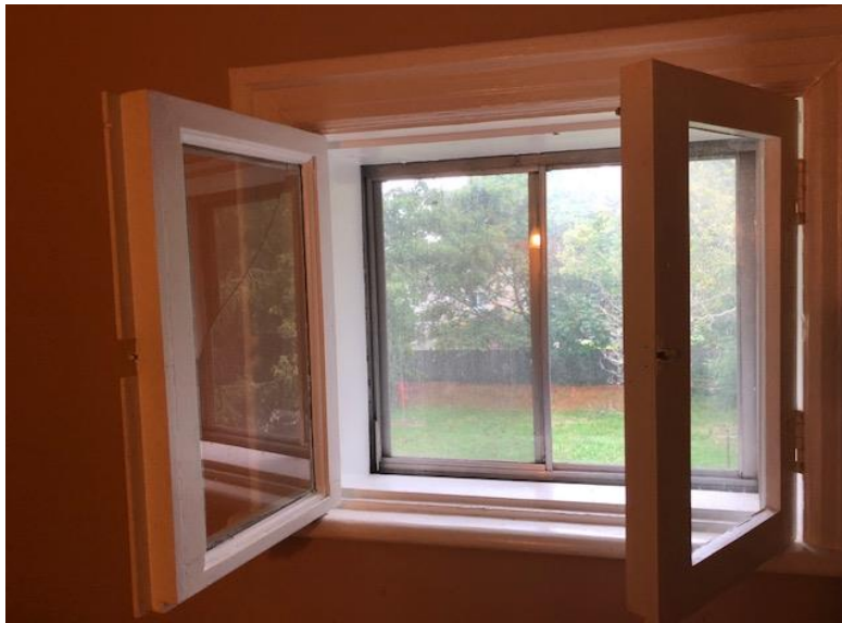
Figure 15: Interior upper floor bathroom window of 22 University Ave. W. Original wood dual window to be maintained.
