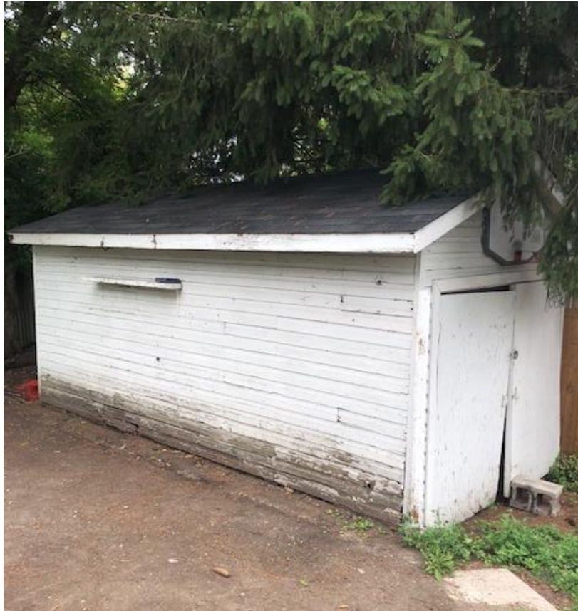
Figure 5: Detached garage to be demolished.
