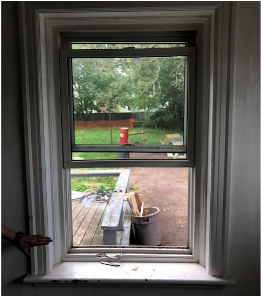
Figure 10: Rear east window of 22 University Ave. W to be replaced (33" x 56") vinyl for vinyl. See product info above. White flashing to be installed approximately where the hand is and across, to allow for a kitchen countertop.
