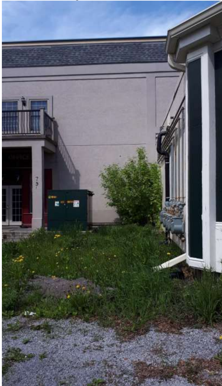
Figure 1: 79 King St. unit E as seen from Third St.
