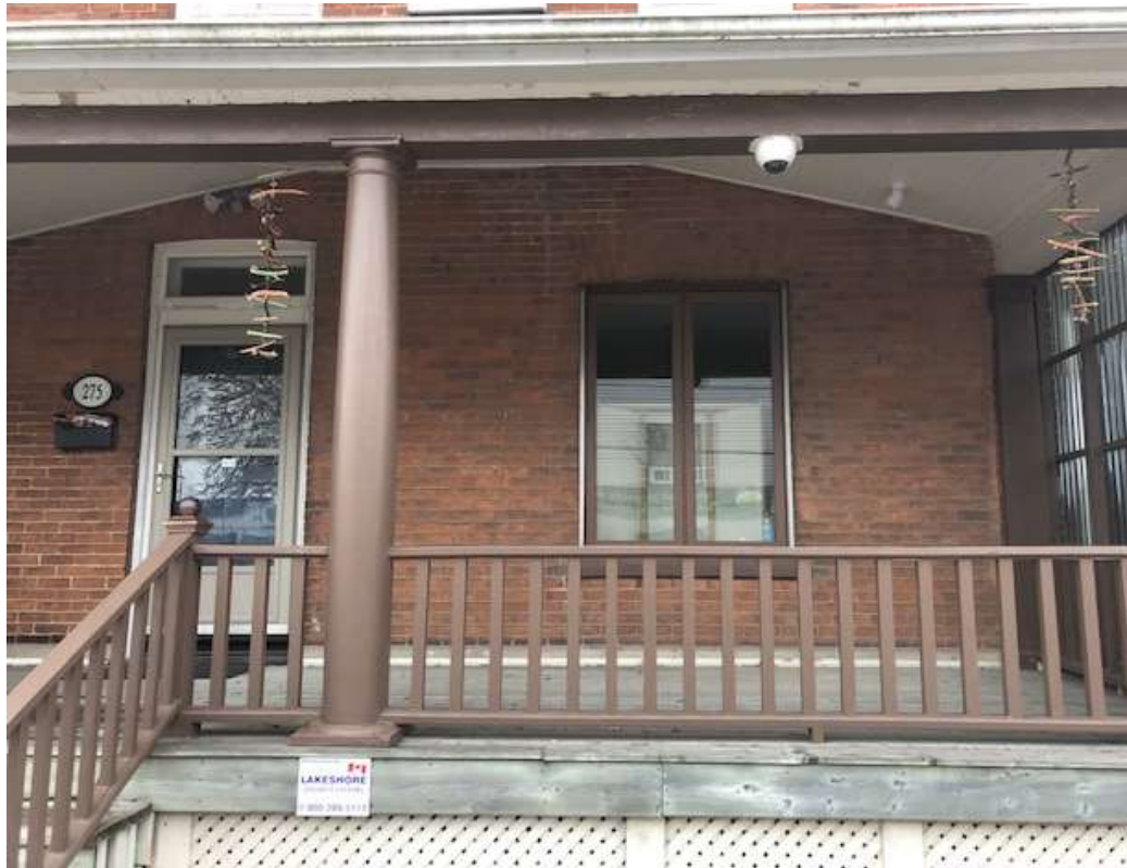
Figure 3: Fall 2018 window alteration to the first floor front window.
