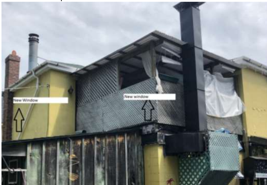
Figure 7: current conditions of 38 Covert St. rear and showing new window placements. Note the covered balcony will be dismantled.
