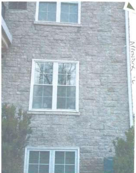
Figure 10: stone façade example (Mansions on George)
