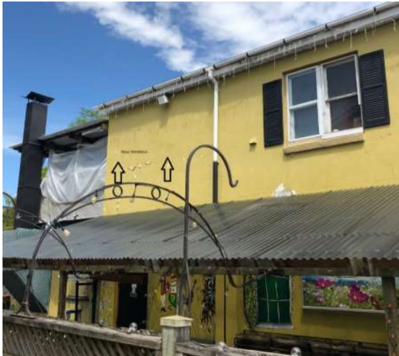
Figure 6: current conditions of 38 Covert St. west side showing where new windows will be placed.
