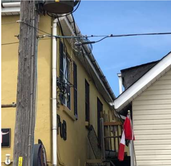
Figure 8: Existing windows on the east facade. Note there will be a new fire window placed toward the rear of this east facade.
