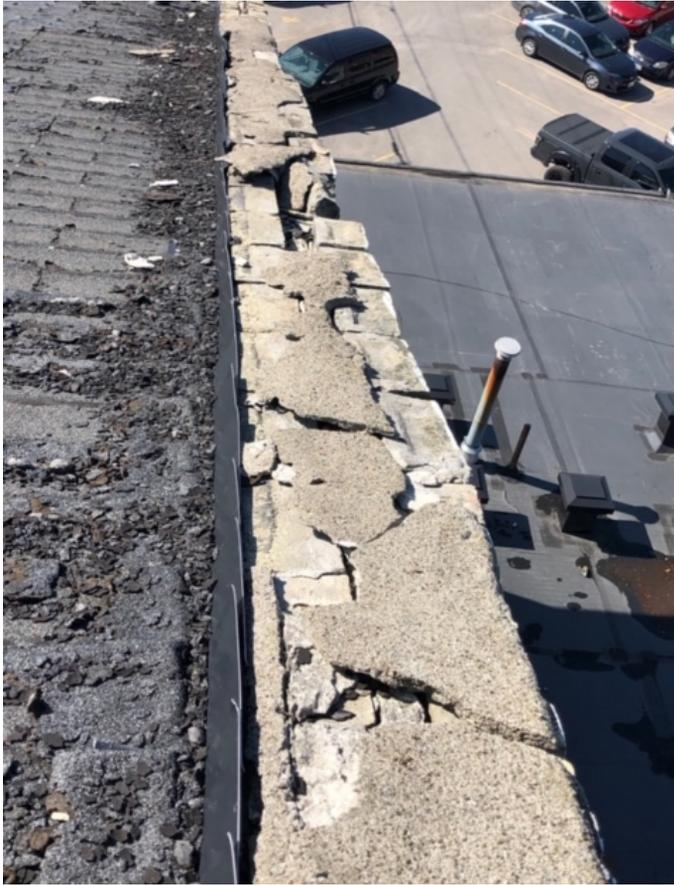
Figure 2: Existing roof, looking west – notice the condition of the partition wall.
