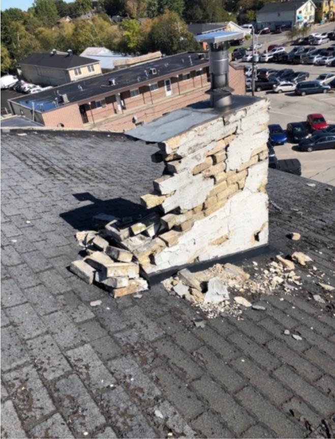
Figure 3: Existing roof – showing existing chimney -- to remain and be rebuilt
