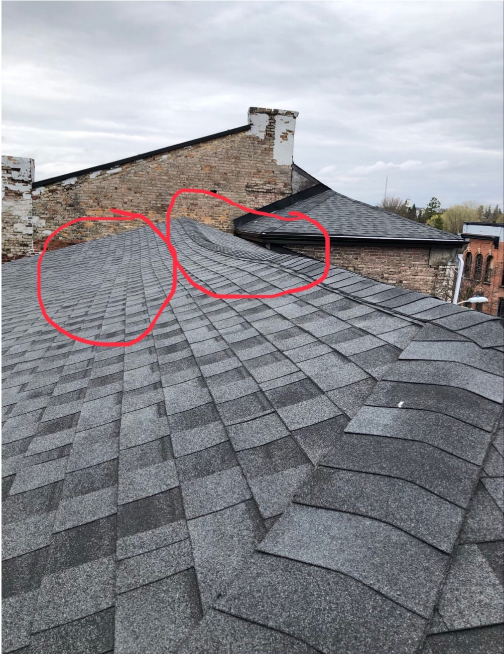
Figure 8: indicating the warping of the roof – to be repaired
