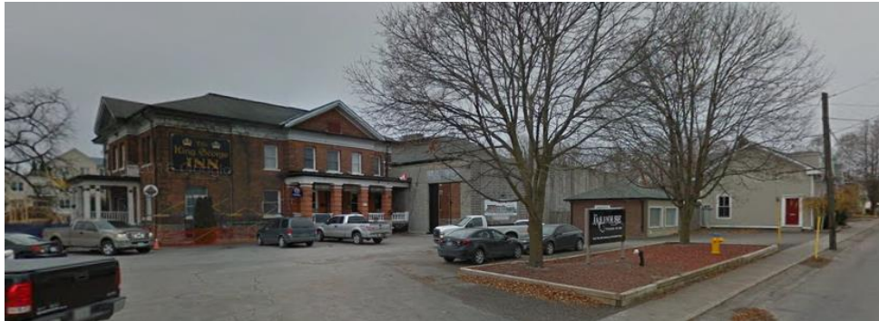
Above: 77 Albert St., as seen from Albert St. looking south
