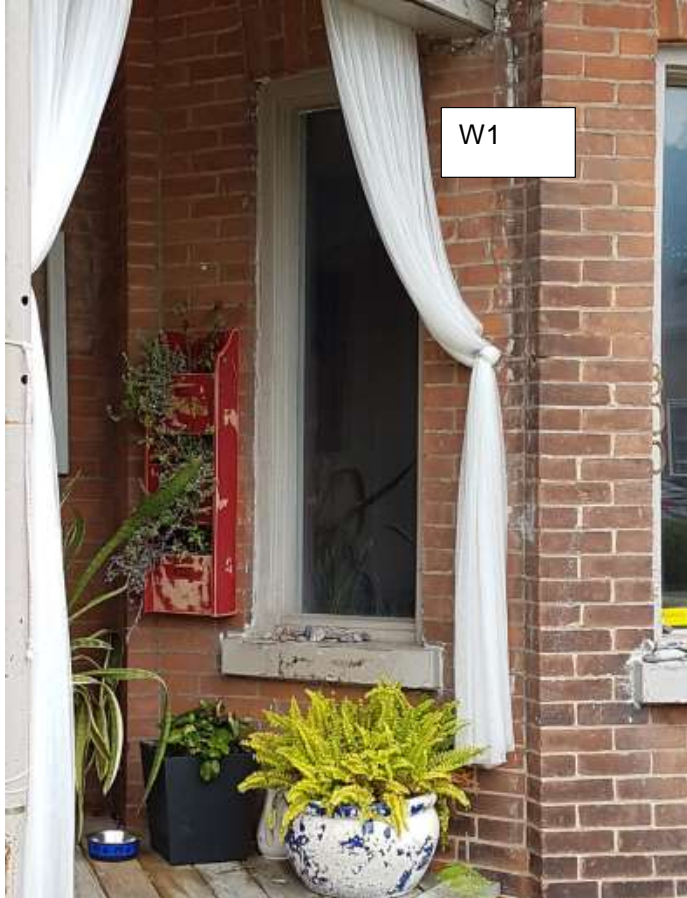
Figure 2: Existing conditions of w1. Wood trim to remain and sill to be repaired. Proposed to be replaced with double hung vinyl
