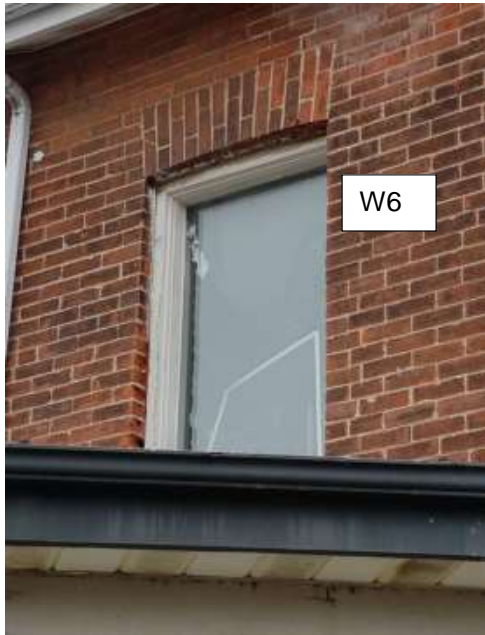
Figure 6: Existing conditions of w6 (upper floor). Proposed to be double hung vinyl. Lintel to remain, wood trim to be maintained and sill to be repaired.
