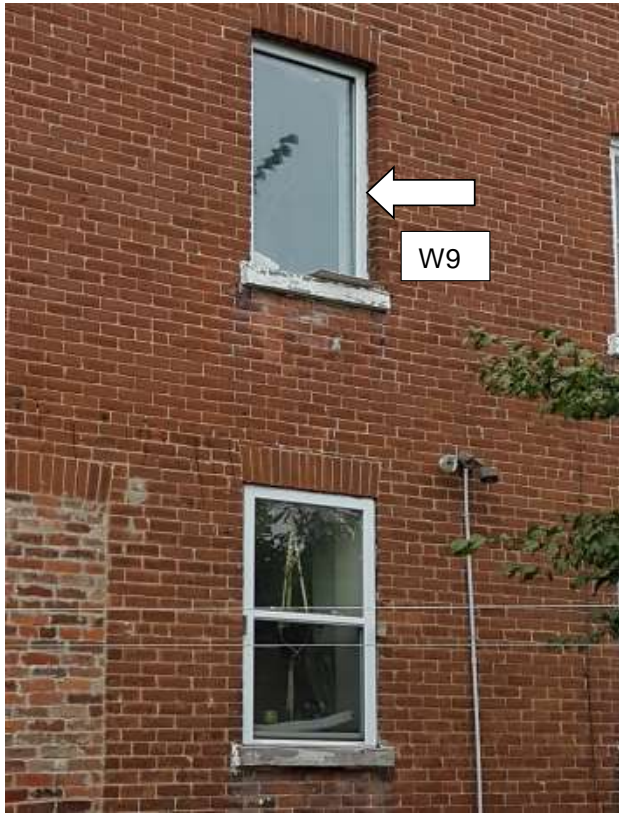
Figure 8: Existing conditions of east-facing w9 (upper floor). Proposed to be double hung white vinyl. Lintel to remain, and sills to be repaired. Main floor vinyl window to remain as is.
