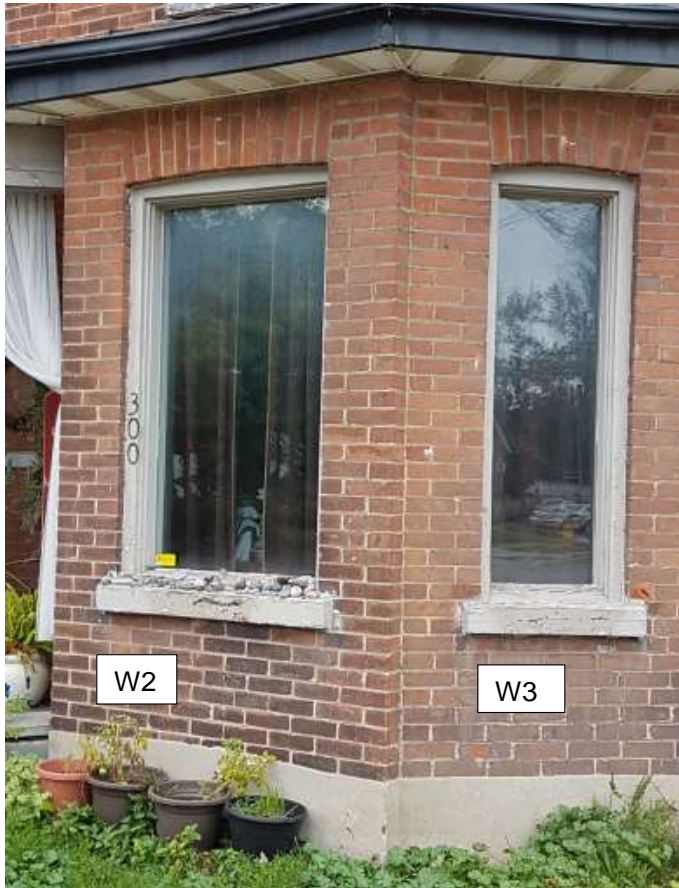
Figure 3: Existing conditions of w2&w3. Wood trim to remain and sills to be repaired. Proposed to be replaced with double hung vinyl.
