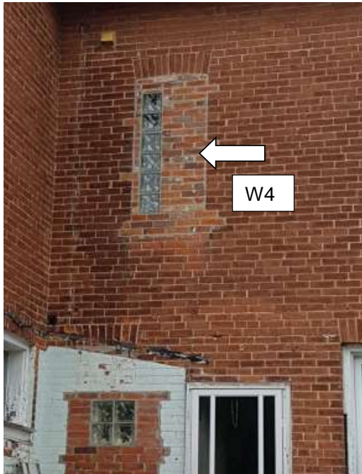
Figure 4: Existing conditions of w4. Notice the glass tile that was installed sometime in the past. Proposed to be double hung vinyl in white. Lintel to be maintained.
