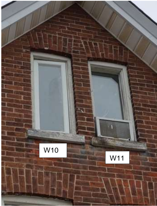
Figure 10: Existing conditions of windows w10 & w11. W10 is currently a vinyl with a broken crank and w11 is seen with an A/C unit installed. Both are proposed to be vinyl double hung in white. Wood trim to be maintained and sills to be repaired.
