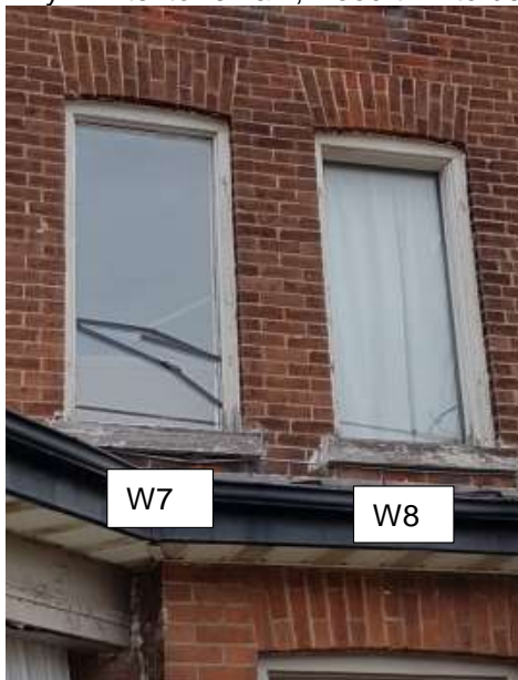
Figure 7: Existing conditions of w7&w8 (upper floor). Proposed to be double hung vinyl. Lintel to remain, wood trim to be maintained and sills to be repaired.
