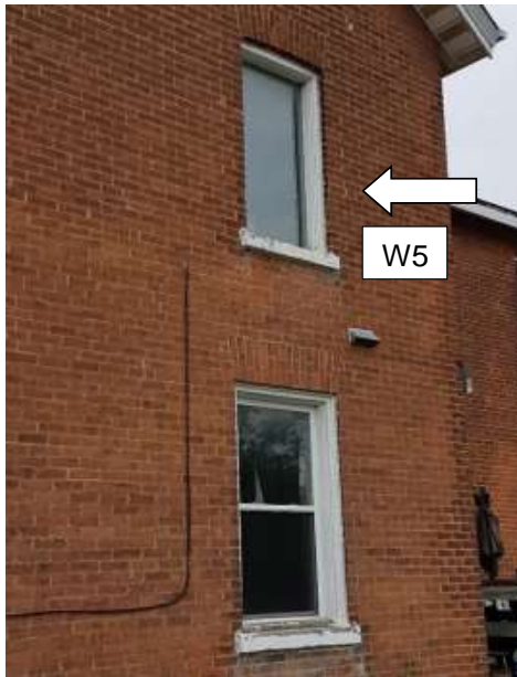
Figure 5: Existing conditions of w5 (upper floor). Proposed to be double hung white vinyl. Sill to be repaired. Main floor vinyl window to remain as is, with sill repaired.
