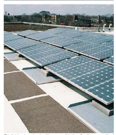
This lightly coloured cool roof has some of the benefits of a green roof and integrates photovoltaic cells to supplement the building energy needs.
