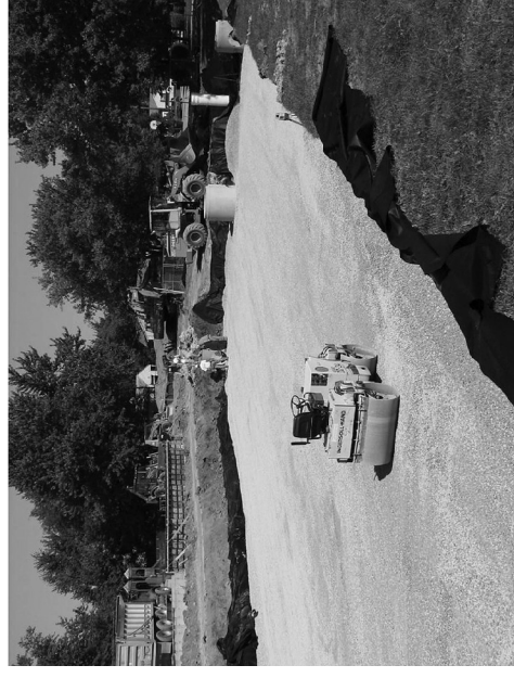
Place clean, crushed, angular stone foundation 6" (150 mm) min. Compact to achieve a flat surface.
