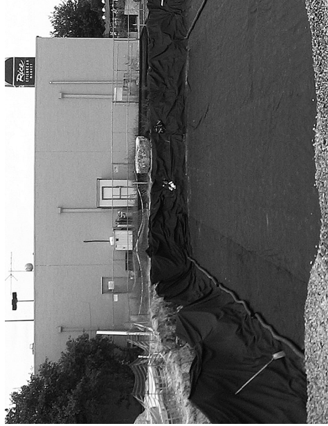
Place non-woven geotextile over prepared soils and up excavation walls. Install underdrains if required.
