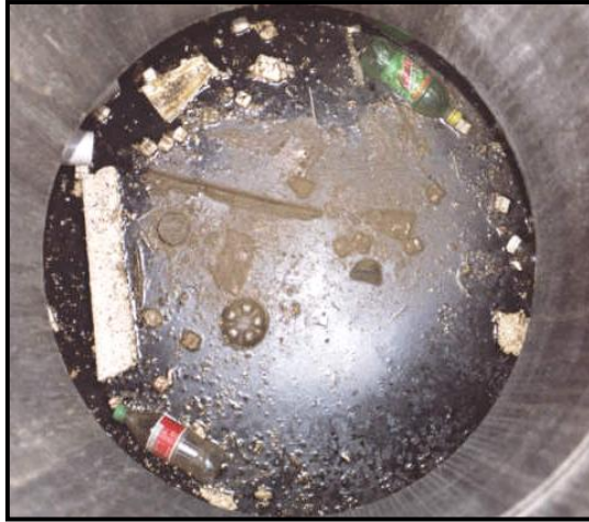
Floatable debris in the Aqua-Swirl®
