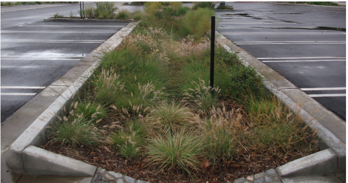
Figure 16: Precedent example of bio-retention area in parking island
