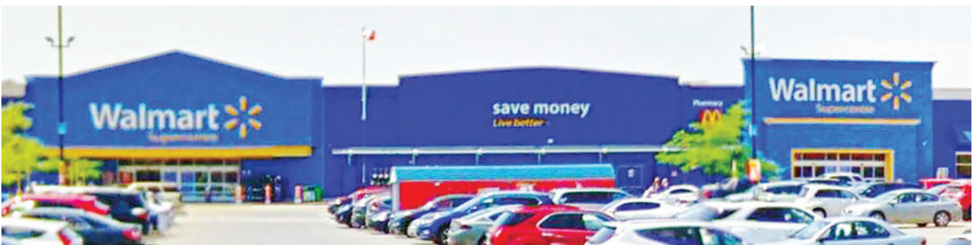
Figure 14: Existing main entrance of Walmart
