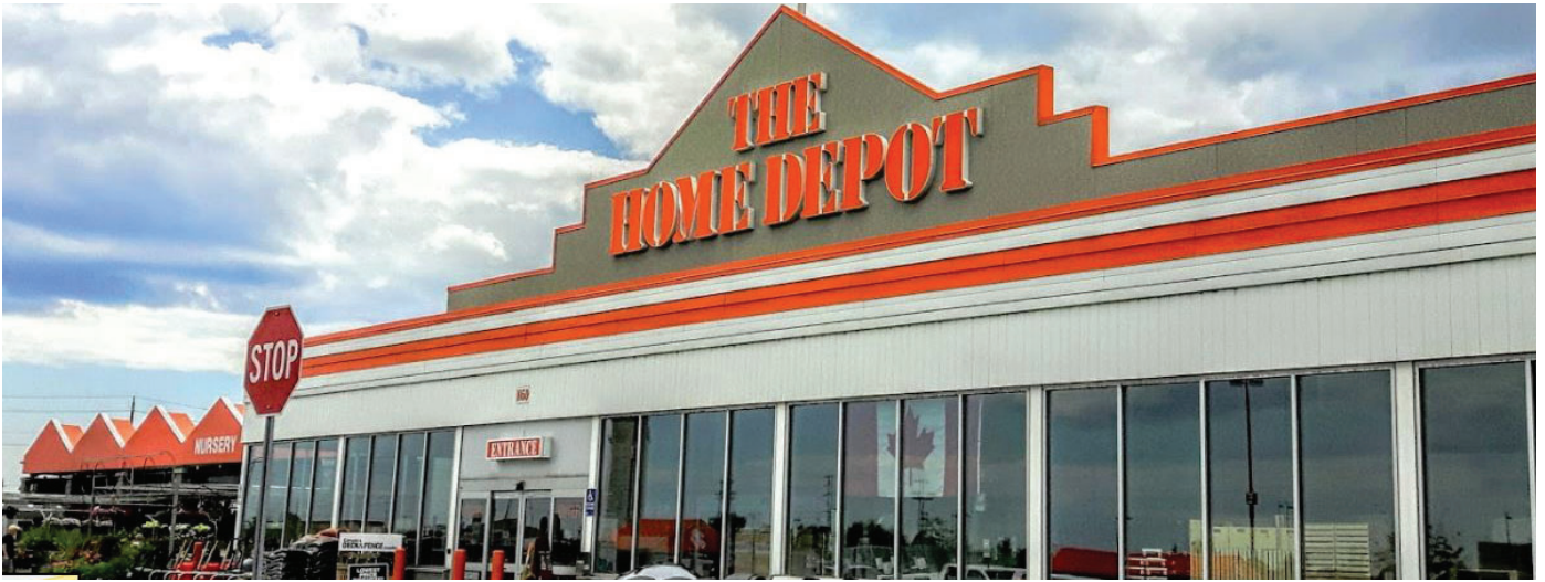
Figure 13: Existing main entrance of Home Depot
