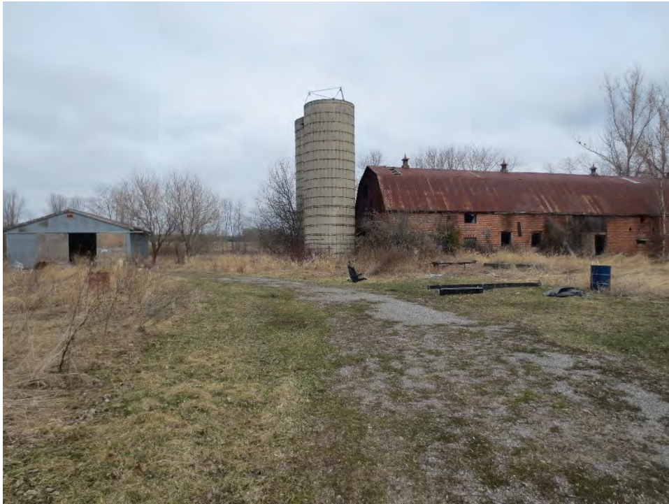
Photo 3 – View of existing barn and work shop near central area of site looking towards the north.
