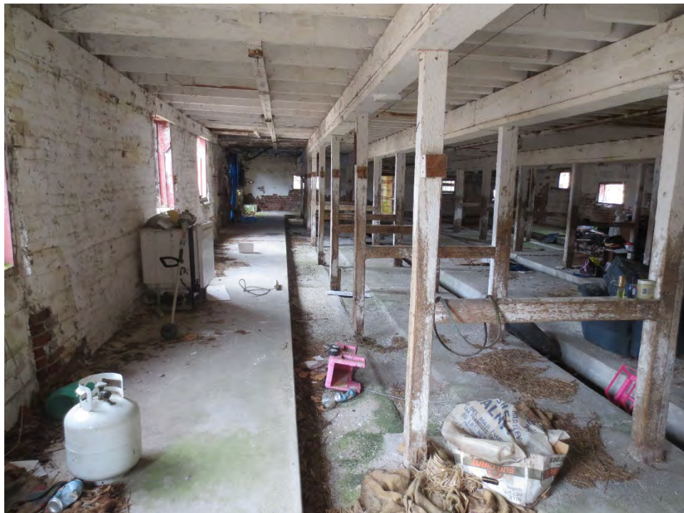
Photo 6 – View of barn interior (typical) looking towards the west.
