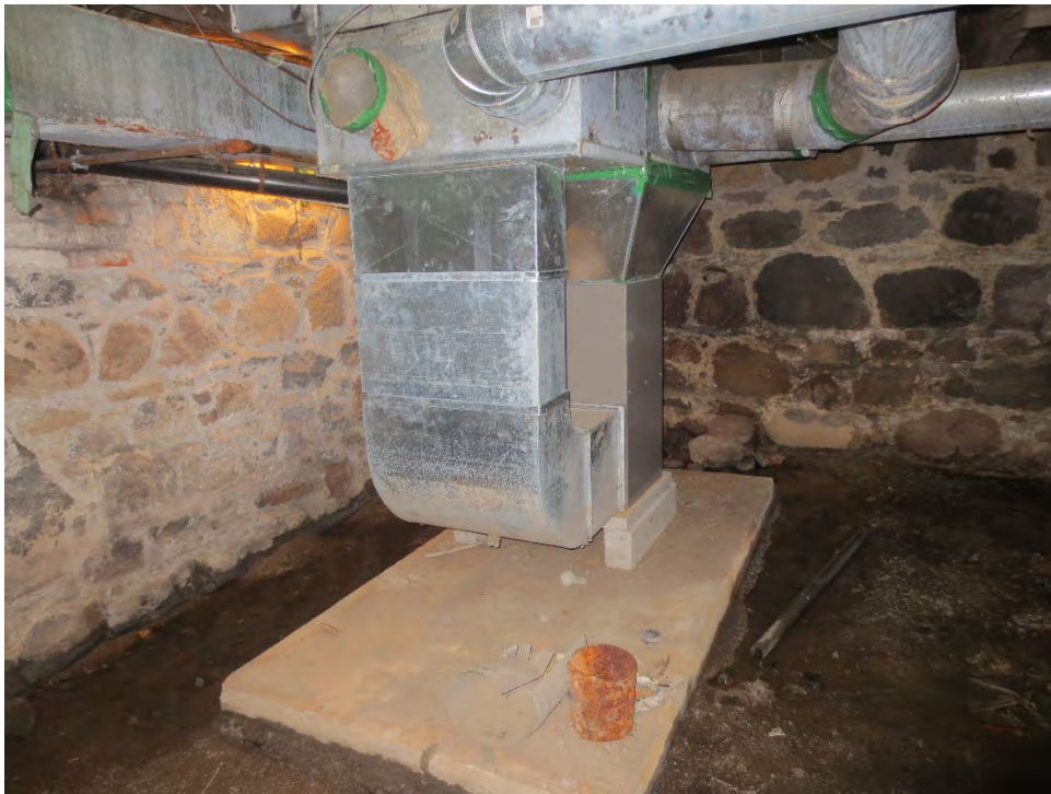
Photo 5 – View of basement area of house (typical) looking towards the southeast.
