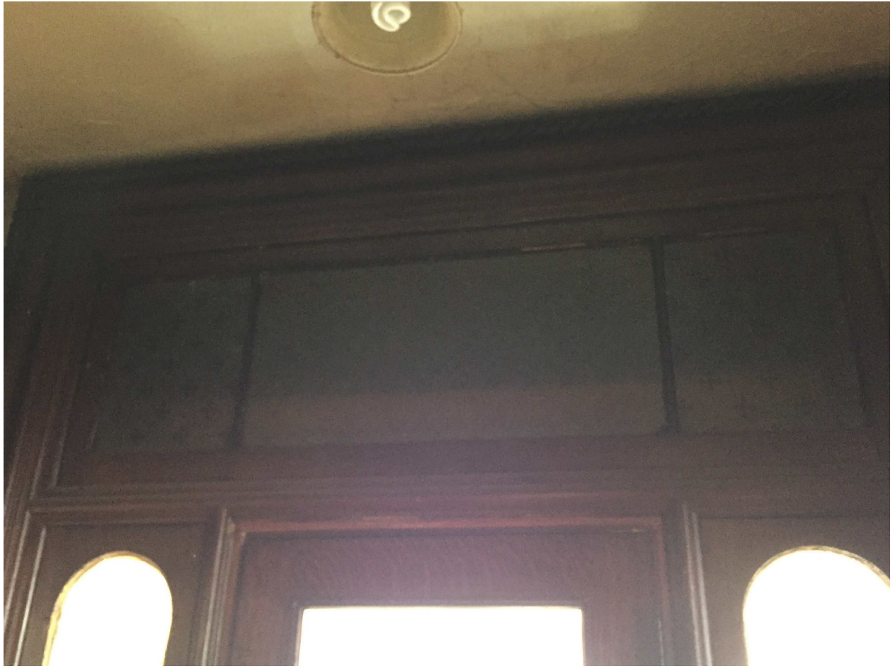
Covered-over front door transom from the inside.
