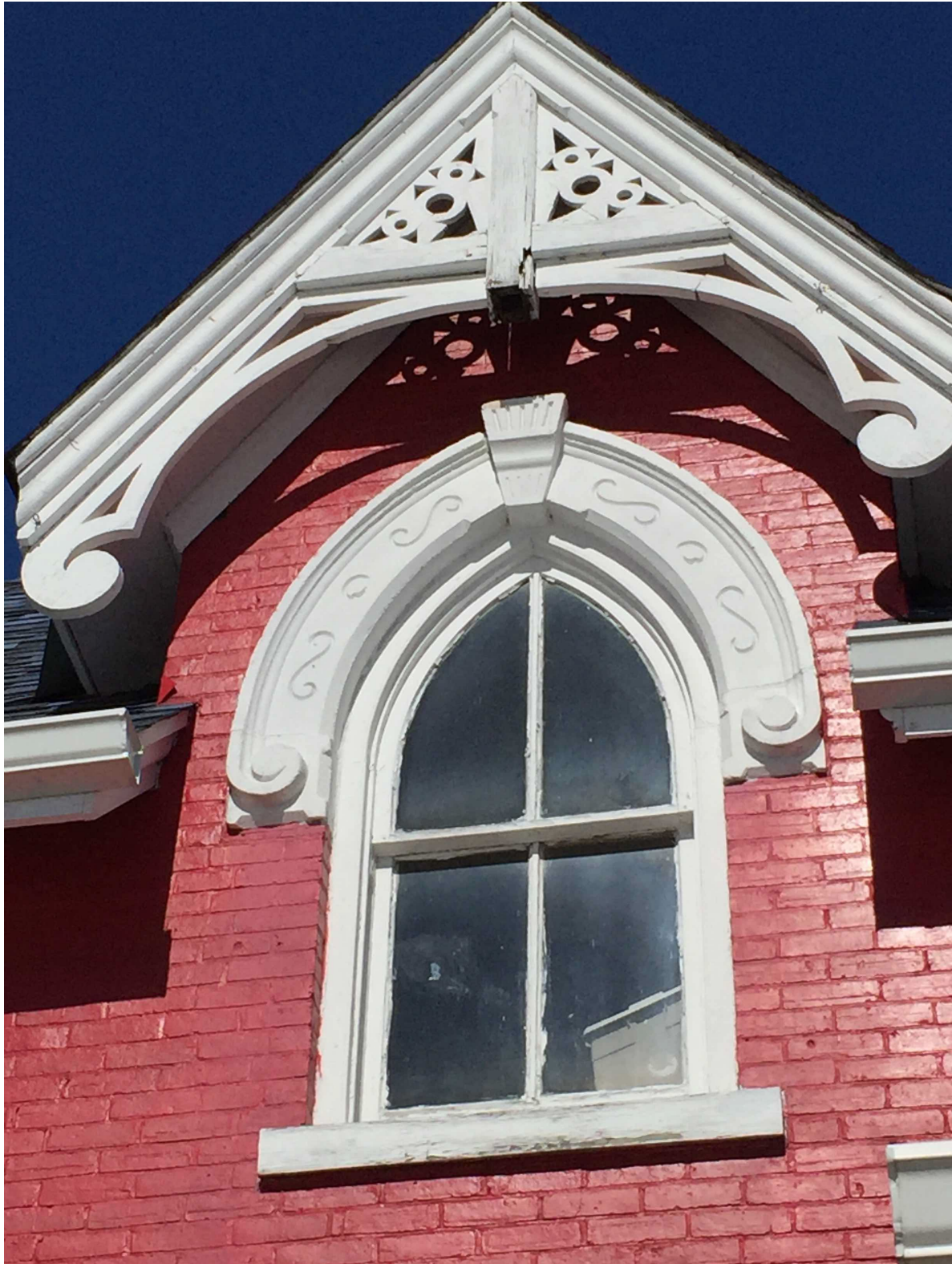
Second-floor dormer with two-over-two lancet window, hood mould, decorative vergeboard, and trusses.
