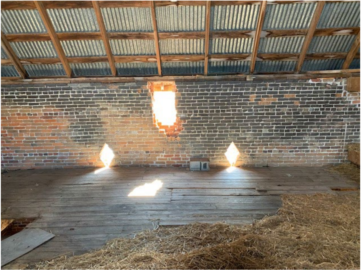
Diamond-shaped openings for light and ventilation
