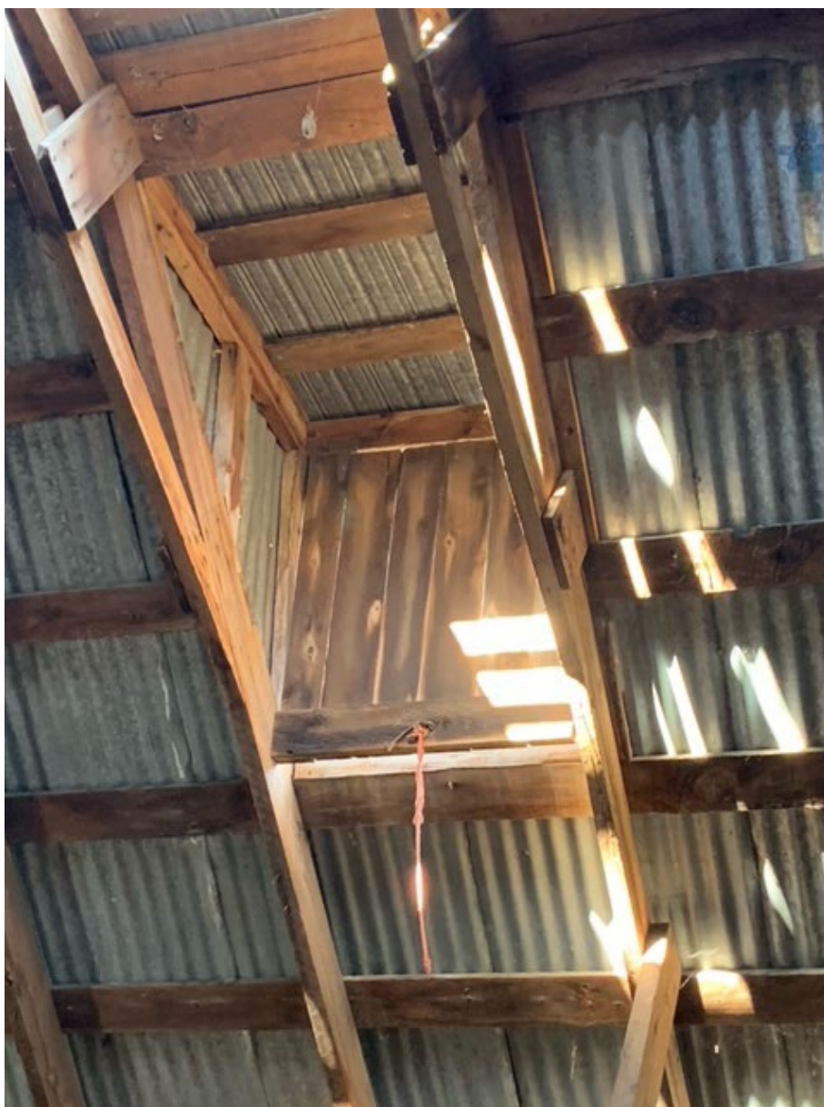
Roof hatch in north elevation
