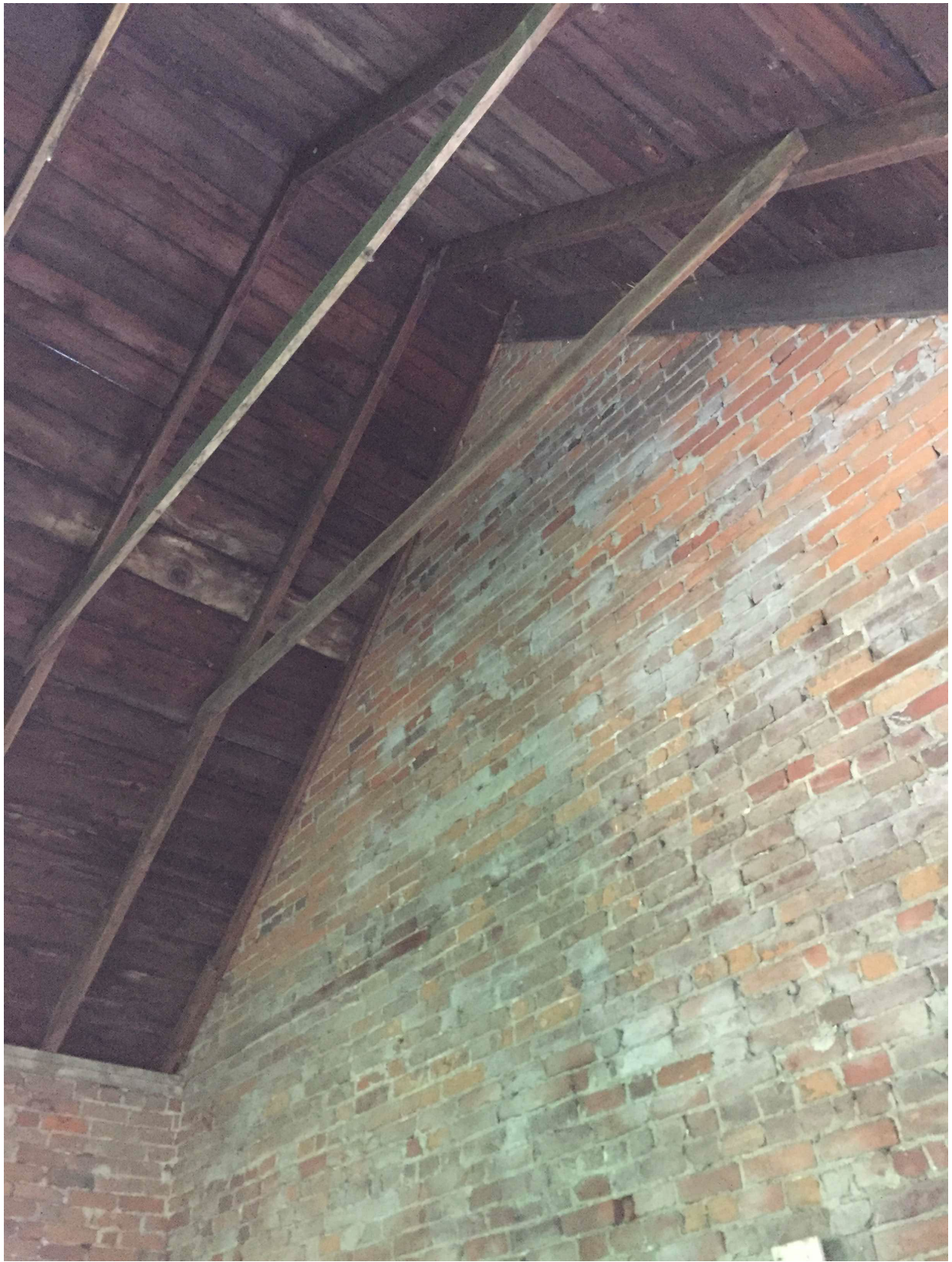
East wall of drive shed from inside
