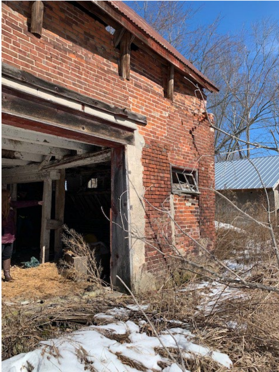
East end addition
