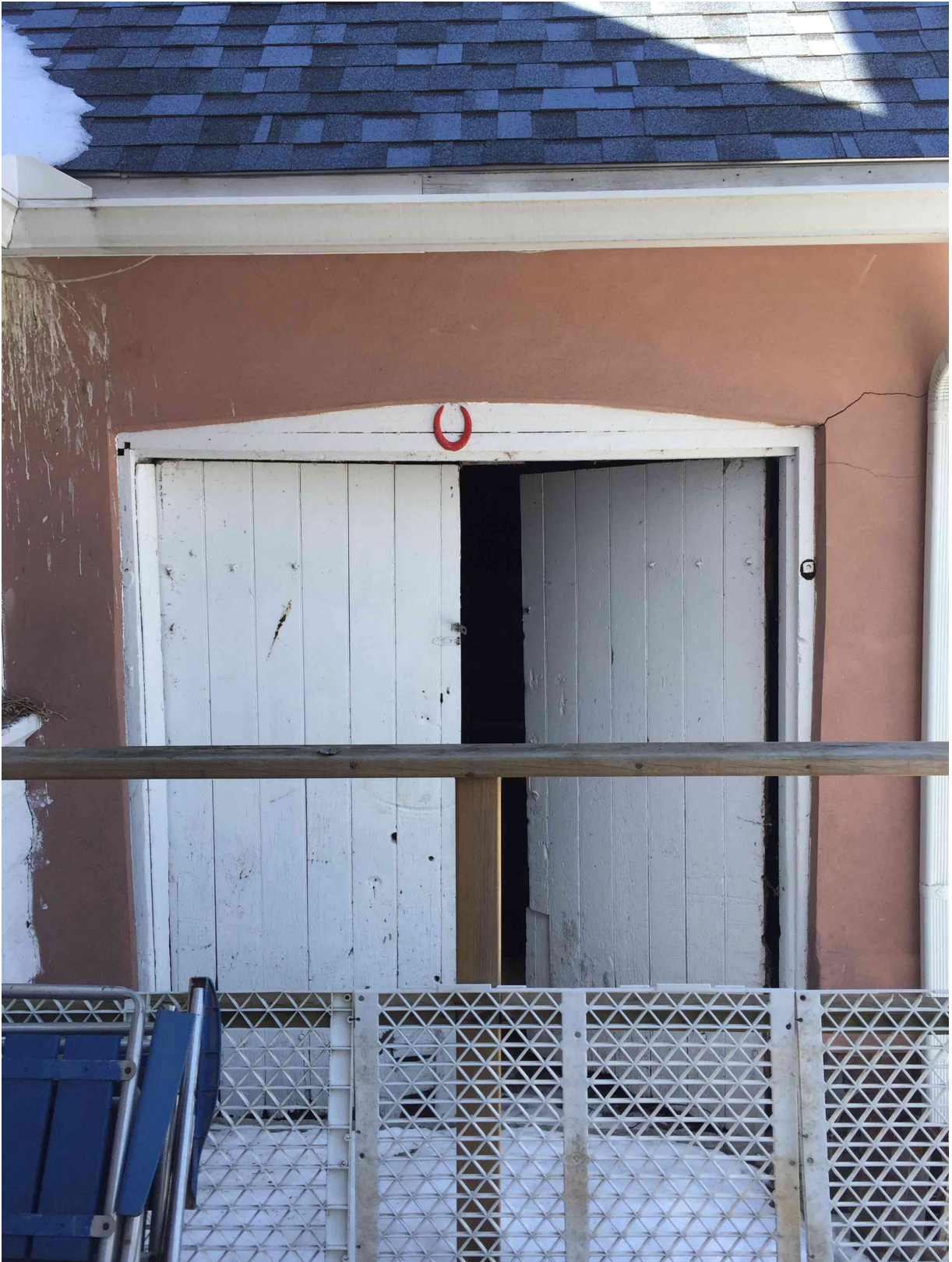
Entrance to drive shed, south elevation
