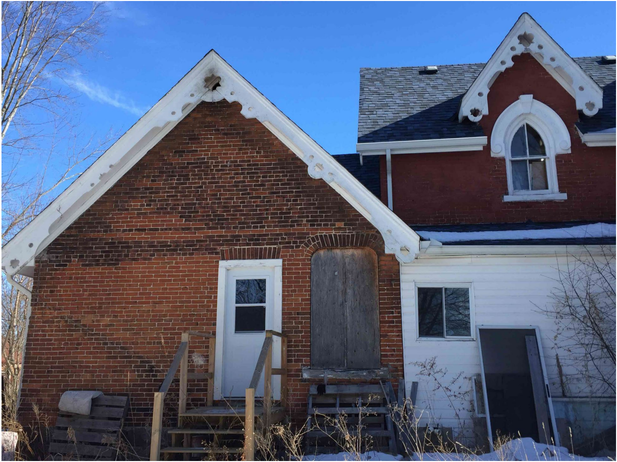
Drive shed, west elevation
