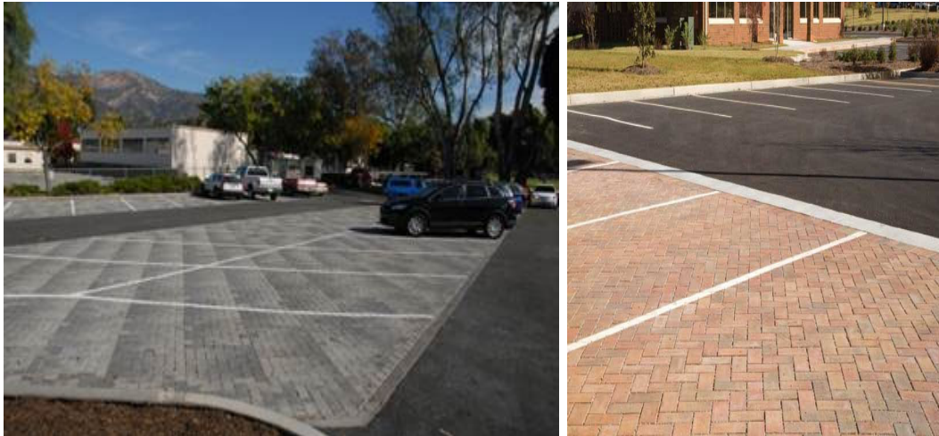
Example of Permeable Pavers and paving patterns
