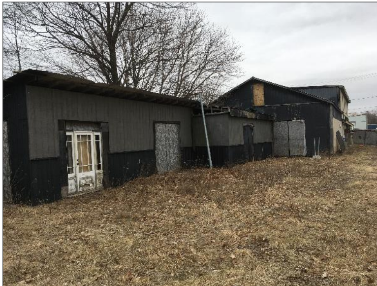
Photo 2 – Site Building A (northeast elevation).
