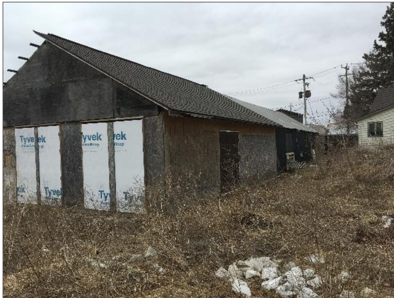
Photo 4 – Site Building B (southeast and northeast elevations).
