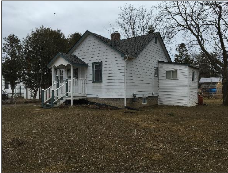
Photo 9 – Site Building E (northwest and southwest elevations).
