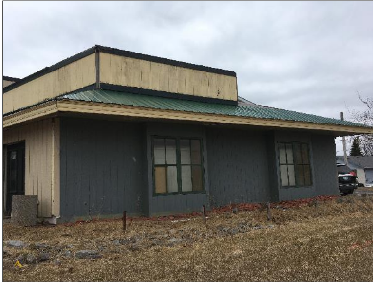
Photo 1 – Site Building A (northwest elevation).
