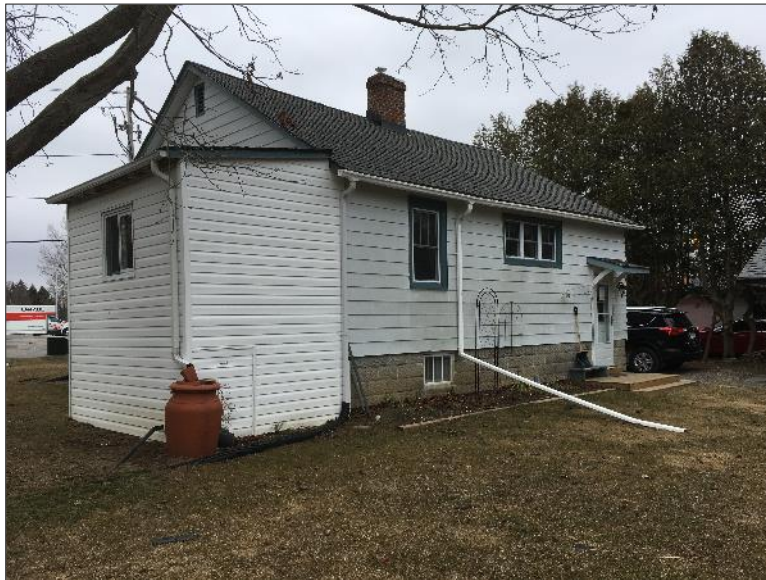
Photo 10 – Site Building E (southeast elevation).
