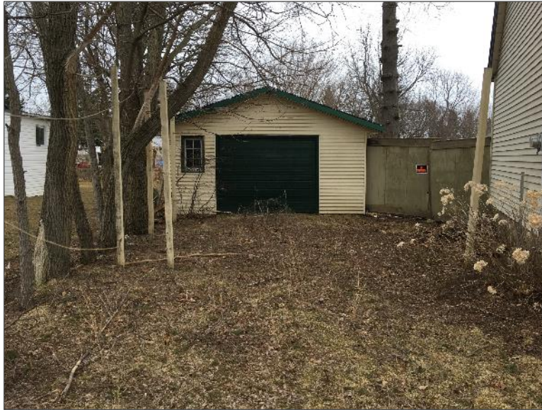
Photo 7 – Site Building D (northwest elevation).
