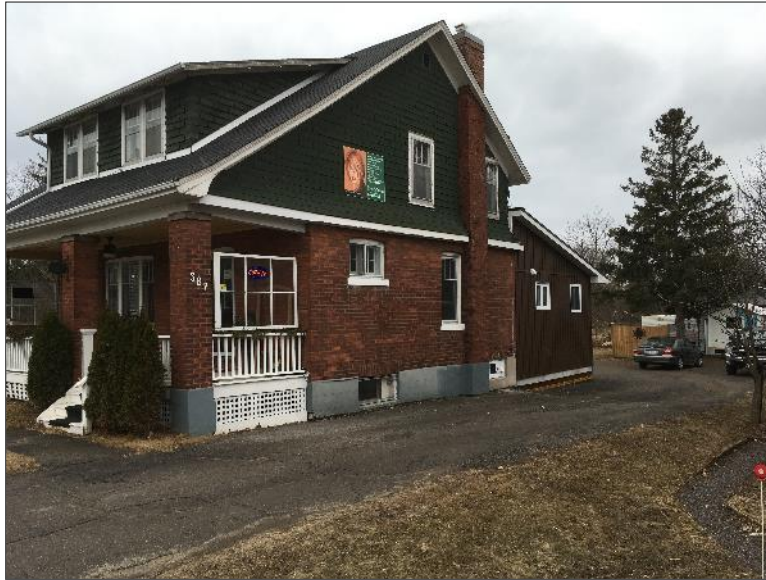
Photo 11 – Site Building F (northeast and northwest elevations).
