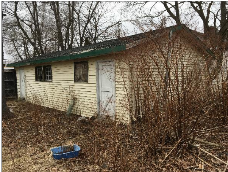
Photo 8 – Site Building D (southeast and southwest elevations).
