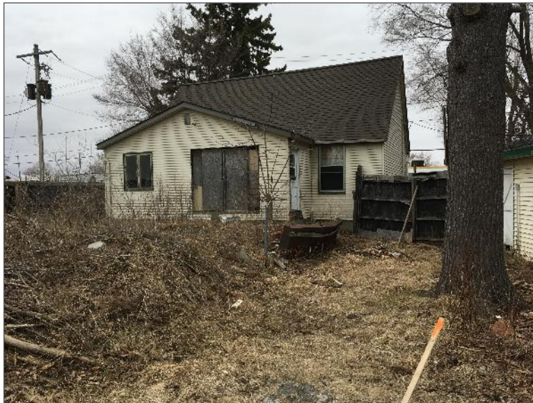
Photo 6 – Site Building C (south and east elevations).
