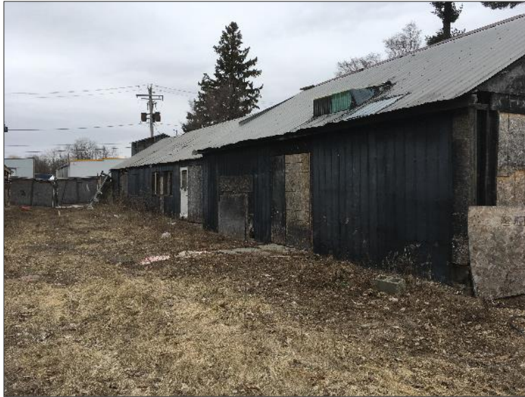
Photo 3 – Site Building B (southwest elevation).
