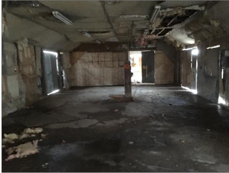
Photo 17 – Interior view of Site Building A.
