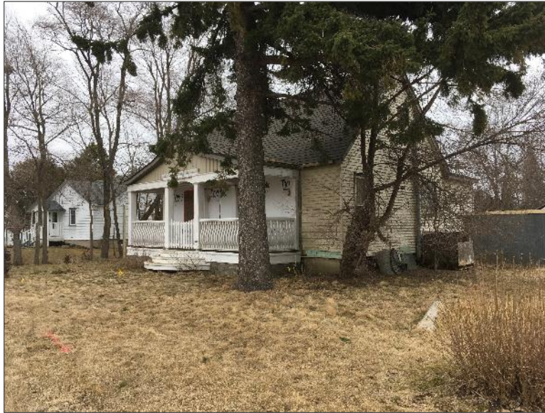
Photo 5 – Site Building C (north and west elevations).
