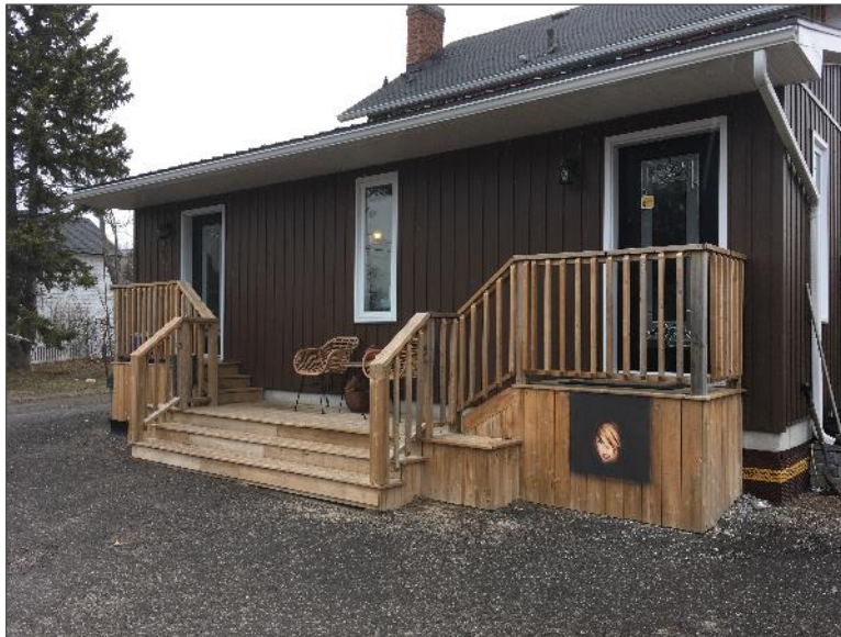
Photo 12 – Site Building F (southwest elevation).
