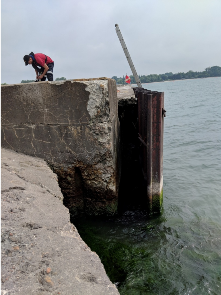
Photo 7 - South End of Pier East Sheetpiles
