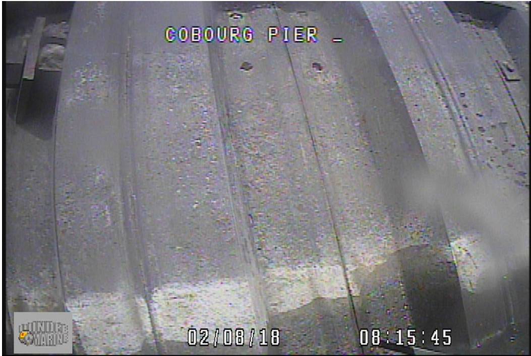
Photo 5 - Tie Rod Bolts Missing East Wall
