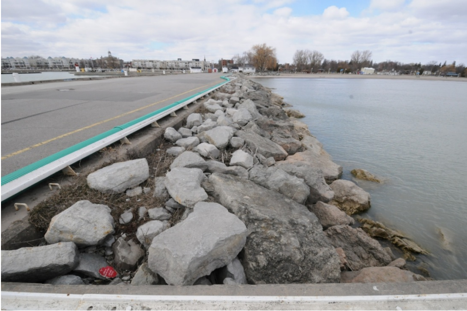
Photo 1 - Revetment East Side
