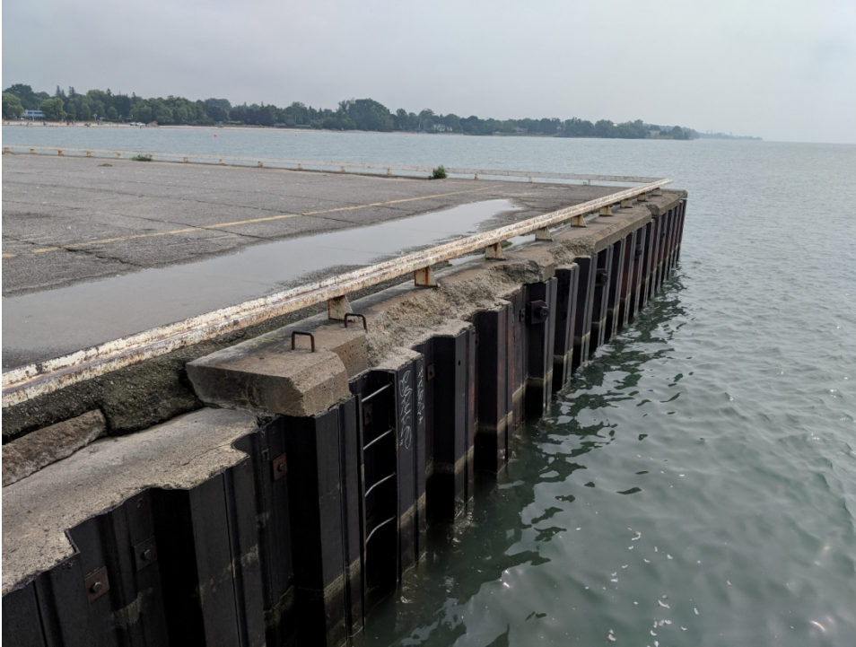
Photo 3 - Deteriorated Concrete Cap Chainage 0+150
