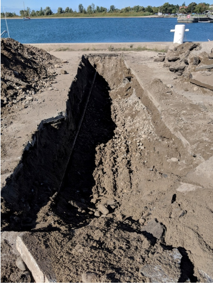
Photo 15 - South Trench Looking West
