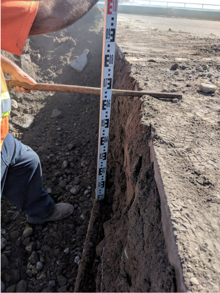
Photo 13 - South Trench Tie
