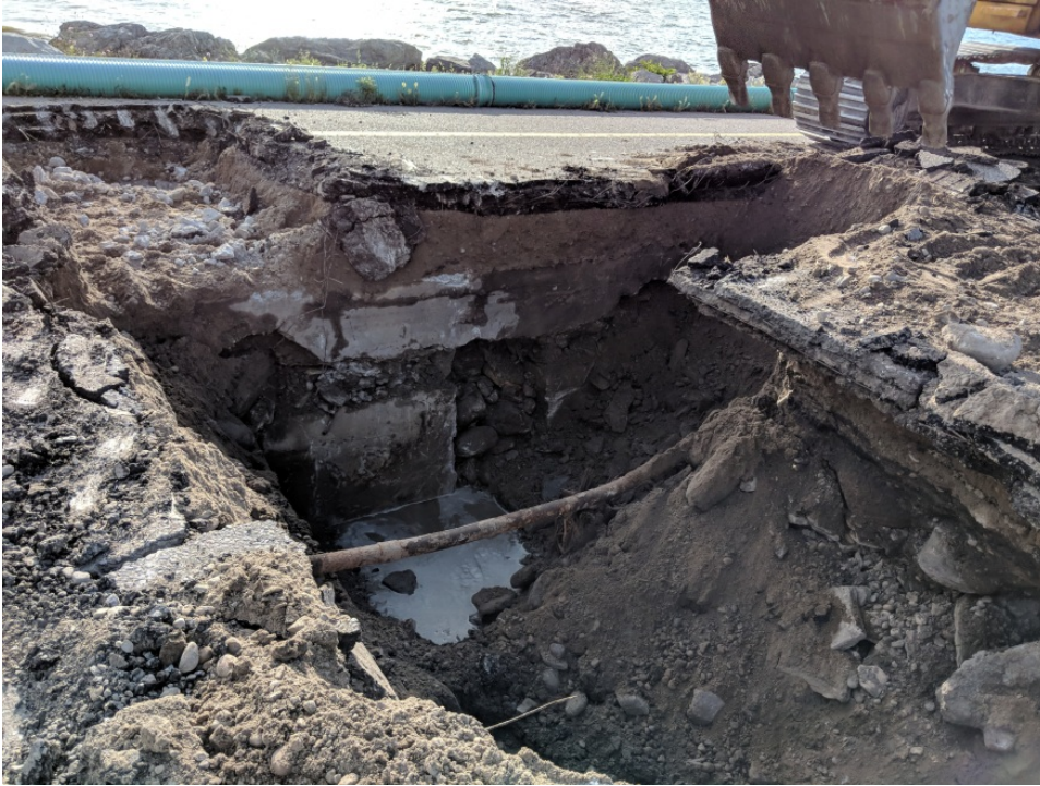
Photo 17 - North Trench Looking East
