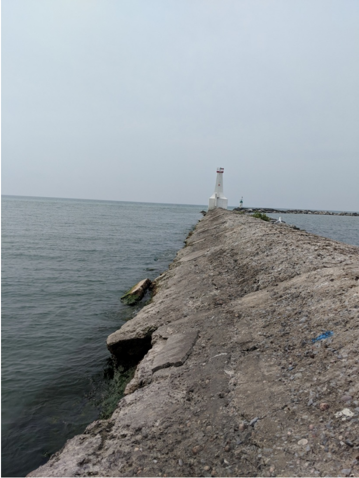
Photo 8 - Concrete Cap Breakwater
