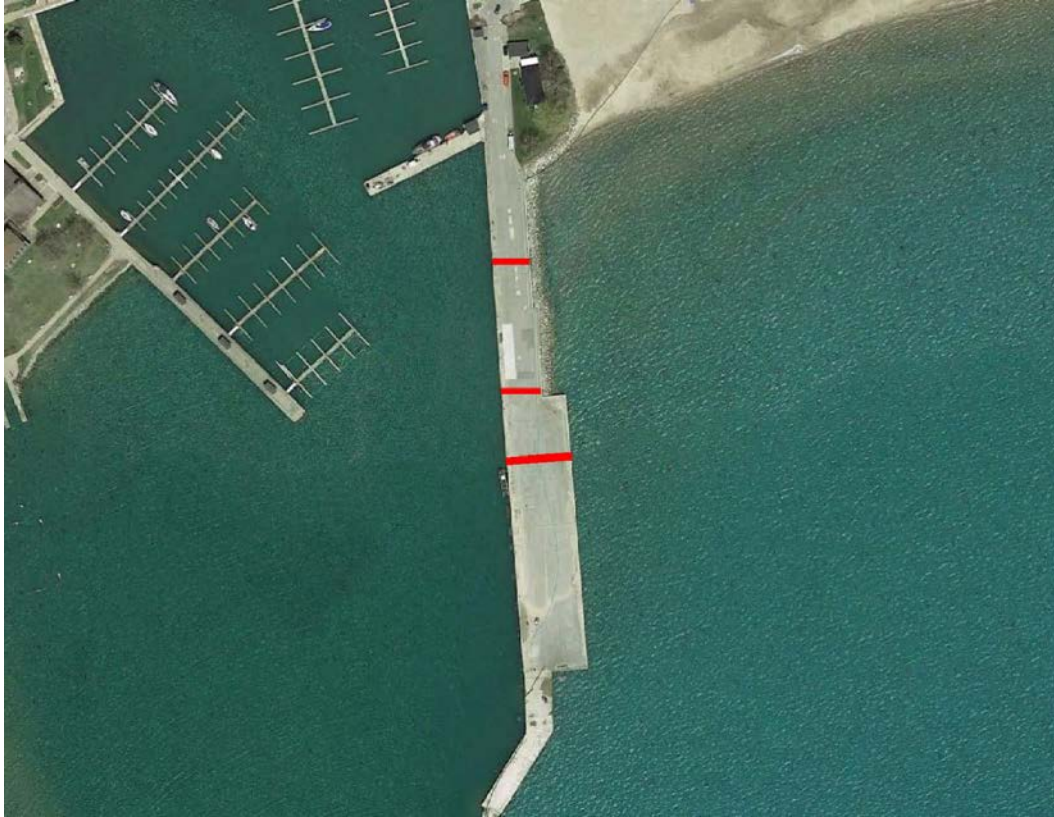
Figure 3 - Test Pit Locations
