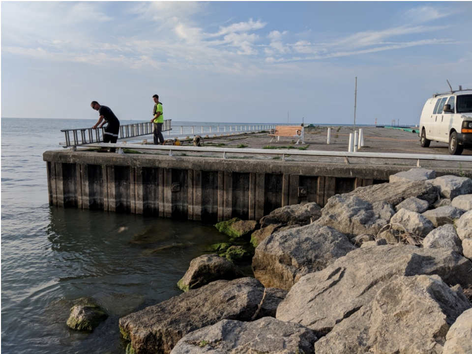
Photo 2 - East Side Steel Sheetpile Wall
