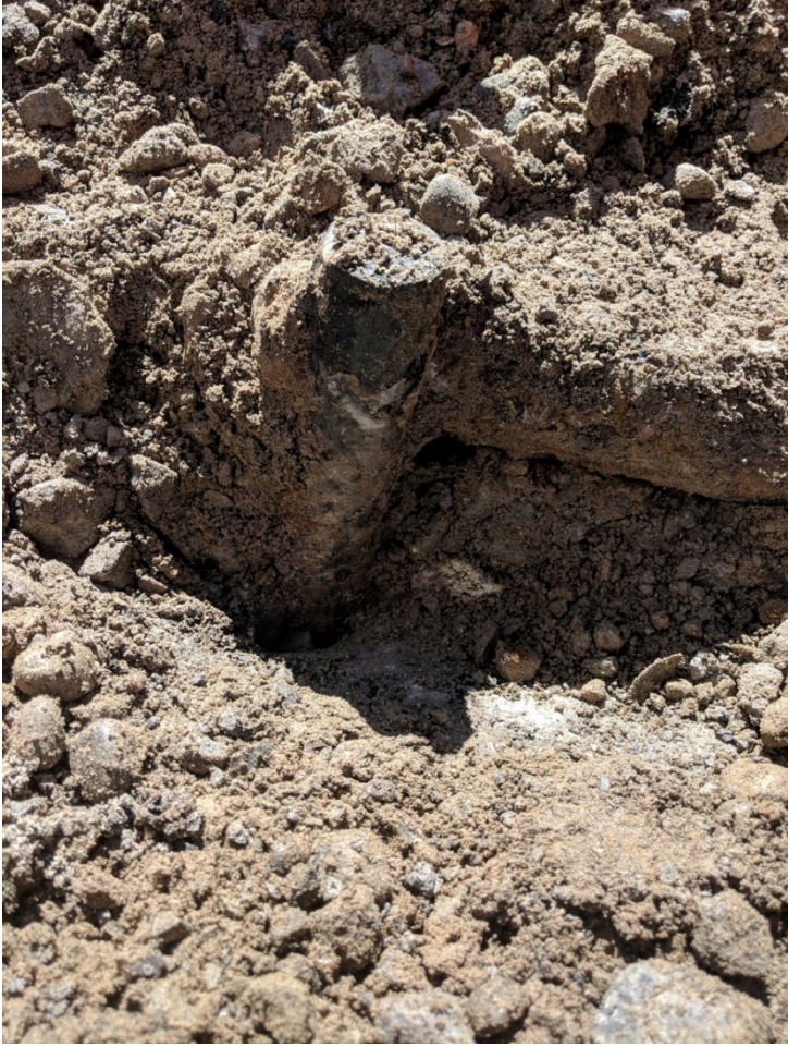
Photo 14 - Pin Holding Tie On Top of Concrete Block
