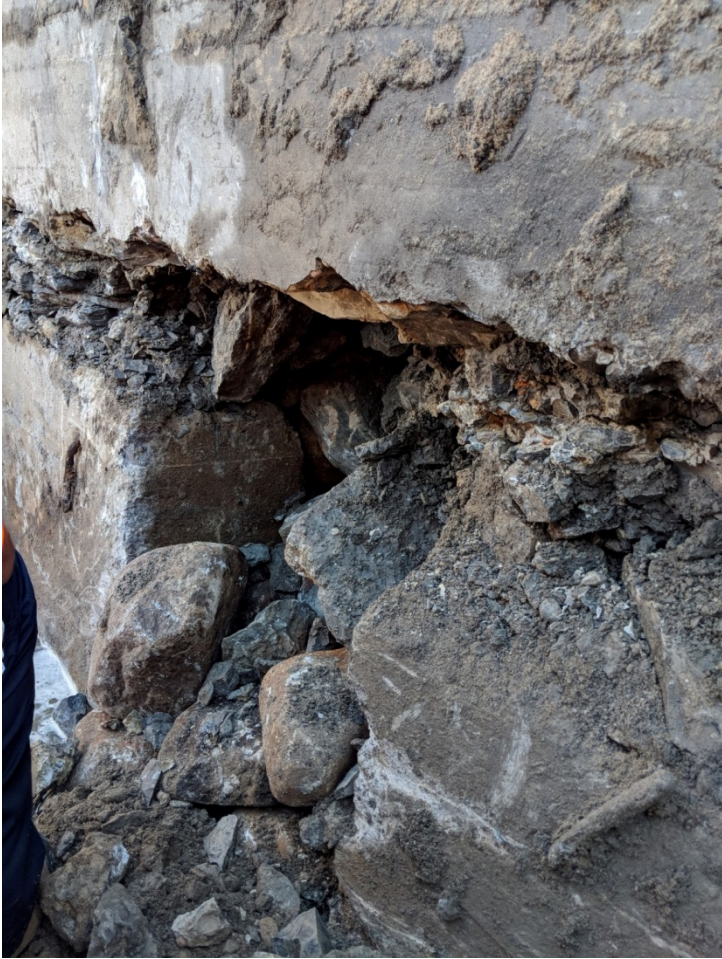
Photo 18 - North Trench Large Stone Fill Without Sand
