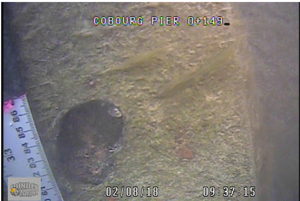
Photo 6 - Cut Hole in East Wall
