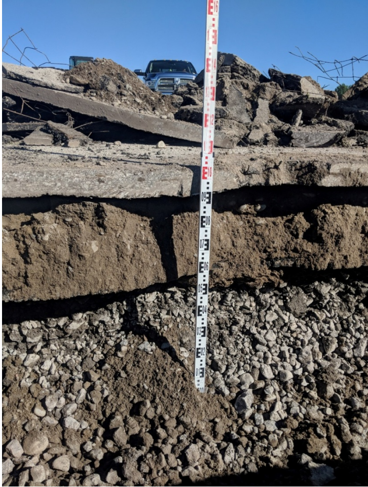
Photo 12 - Double Layer of Asphalt
