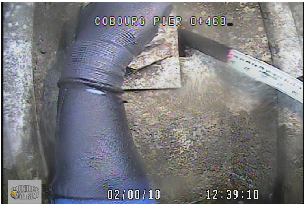
Photo 11 - Tie with Small Hole Beside West Wall
