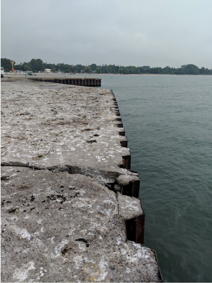
Photo 4 - South End Sheetpiles Without Concrete Cap
