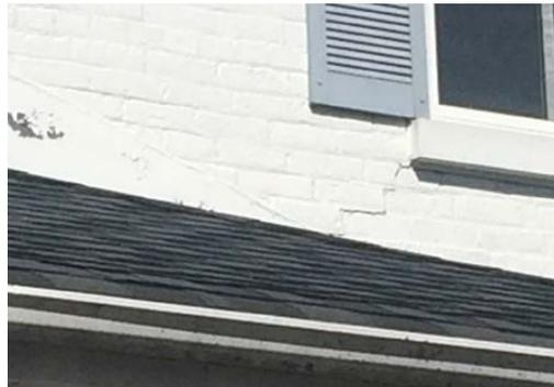
11. Peeling paint and step cracking at side elevation (left) and step cracking at front elevation above porch (right), 2018 (BA)
