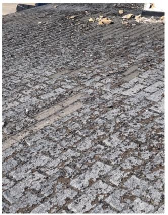
Figure 1: Existing roof – notice the condition
