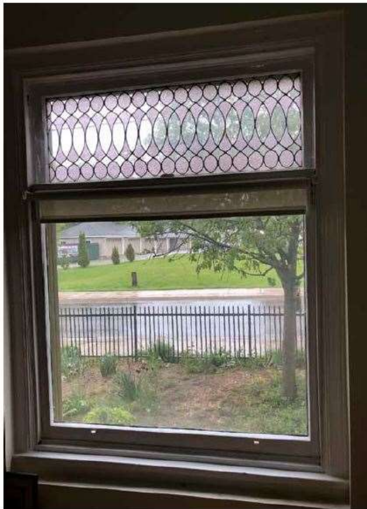
Main front window from inside. Currently will not open. Sash cords are broken.
