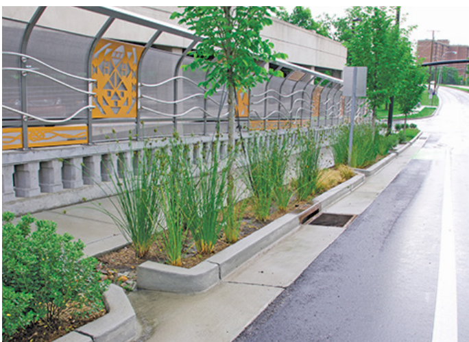
Bioswales or rain gardens can be used to reduce surface runoff and provide a transition area between pedestrians and vehicles.
