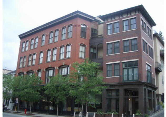
Precedent example of a newly renovated historic mixed use building.
