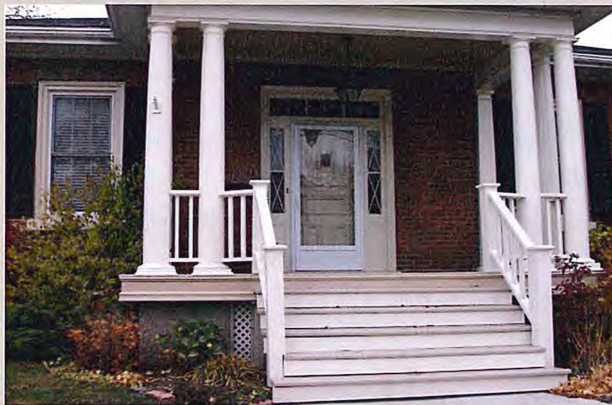
This newly constructed porch was painted with colours from the Cobourg Heritage Palette.
