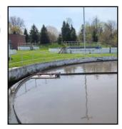
Primary Treatment: The flow enters the Primary Clarifier where the velocity is slowed to allow solids to settle to the bottom and grease to the float to the top. Solids and grease are pumped into the Anaerobic Digester to be converted into Biosolids.
