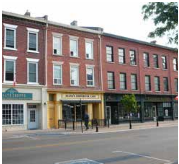
Maintain a consistent built form pattern along commercial streets - view along King Street West, Cobourg.
