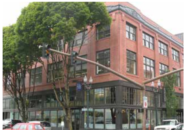
Example of historic façade pattern.
