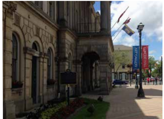
View towards Victoria Hall, Cobourg, Ontario.
