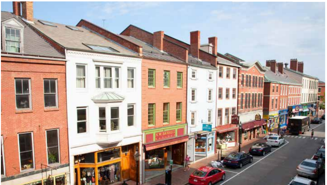
Example of consistent façade design and articulation along a commercial main street.
